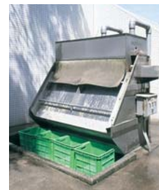
Site: Fish processing plant
