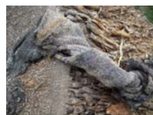
Grinder pump clogging with rags
