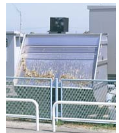
Site: Pump station (River water intake)
