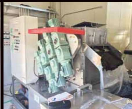
Mixed Sludge at Confectionary Plant (JD-500)
